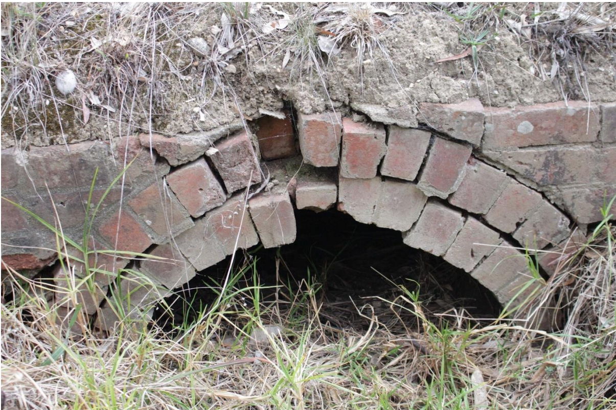
Brick culvert near Ebdon Station (RBA, June 2024)
