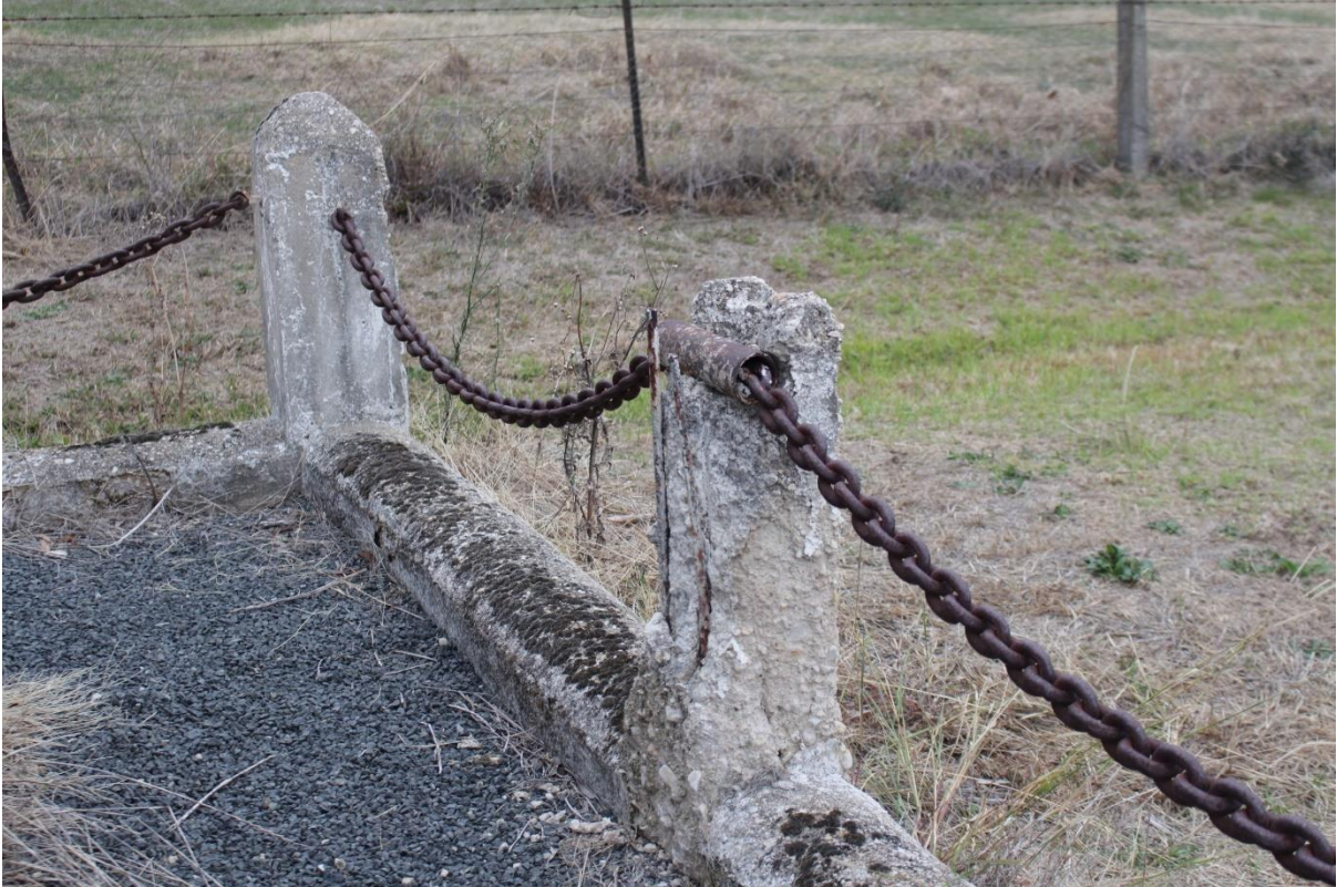
RBA, June 2024 – showing concrete piers and chain
